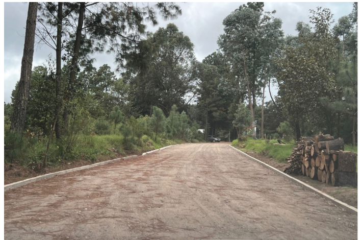
The new road on the property leading to Zeth College
